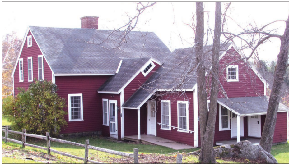
A re-creation of the Hawthorne home is located on the grounds of Tanglewood in Lenox, Massachusetts.
