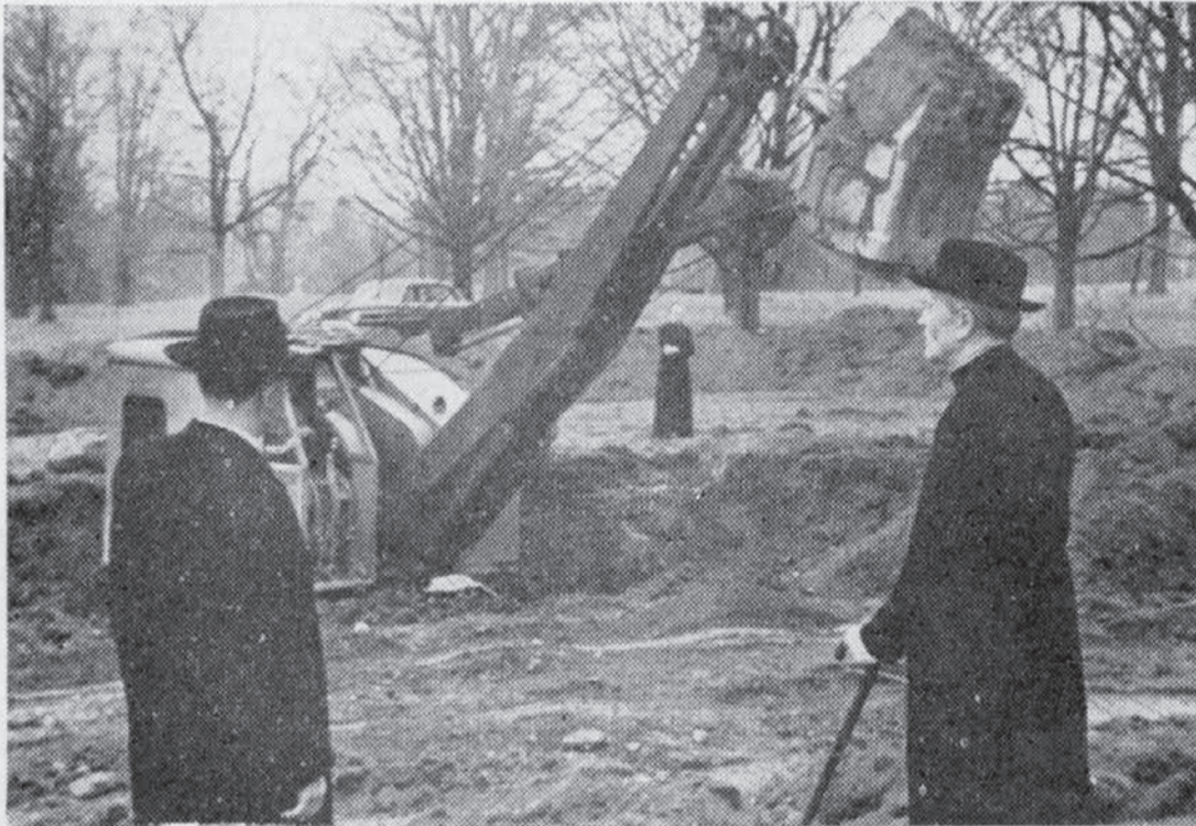
Starting the foundation of our new Chapel
